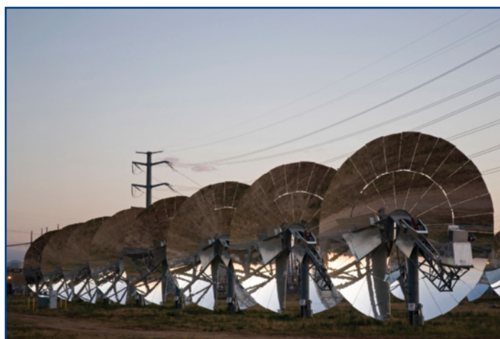
Figure 9.2: Array of parabolic dish solar collectors at Maricopa Solar Project in Peoria, Arizona. The facility consists of a total of 60 parabolic dishes.
