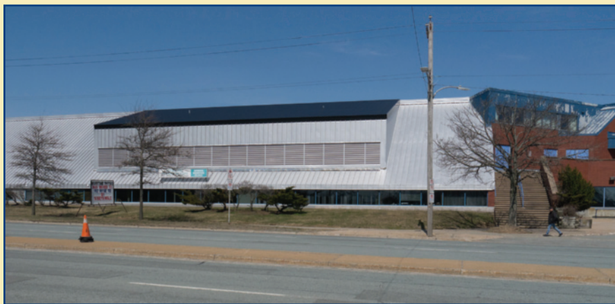
Figure 8.16: Transpired solar collector on the Sportsplex, Dartmouth, Nova Scotia. The 300 m 2 collector is the dark section of the roof near the center of the building.
