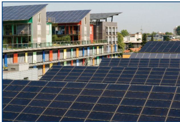
Figure 9.27: Photovoltaic solar panels on homes in the ecological Vauban district in Freiburg, Baden-Wuerttemberg, Germany.
