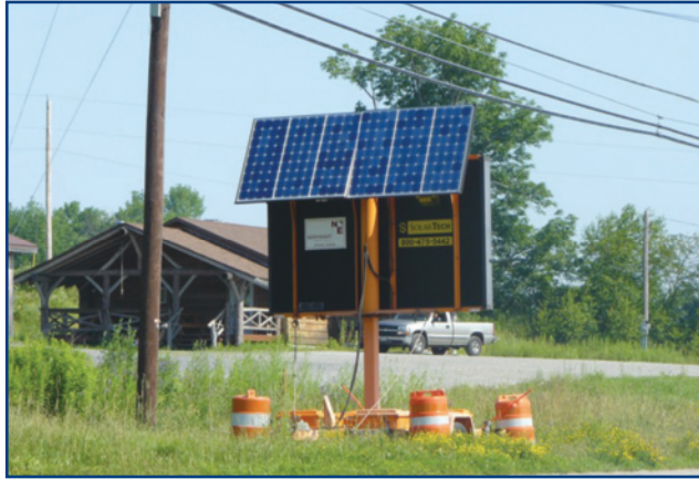
Figure 9.25: Portable road sign at construction site that utilizes a photovoltaic array (about 1\text{ m} \times 2.5\text{ m} ) to charge batteries.
