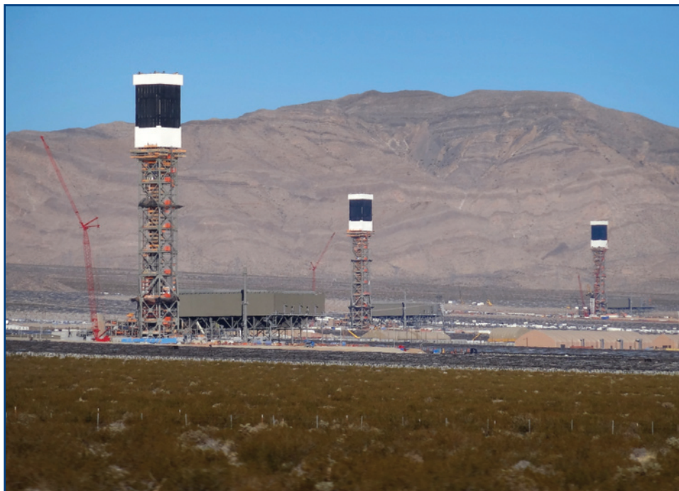
Figure 9.8: Three collector towers at the Ivanpah Solar Electric Generating Station in the Mojave Desert in California.
