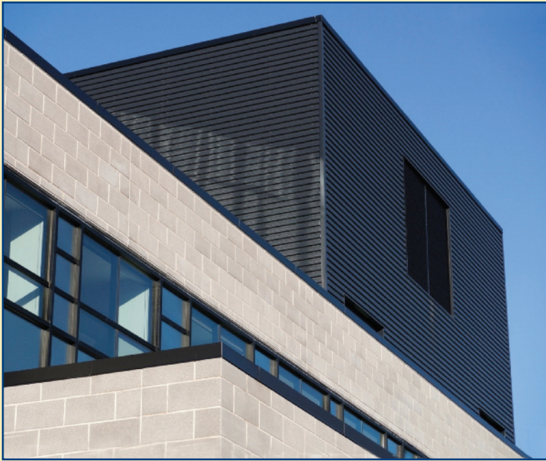
Figure 8.15: Transpired solar collector on the south- and west-facing walls of the Mona Campbell Building at Dalhousie University, Halifax, Nova Scotia, Canada. This building has LEED Gold certification (see Energy Extra 17.1).
