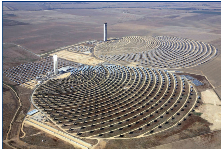
Figure 9.7: The PS10 rated at 11 MW e (foreground) and PS20 rated at 20 MW e (background) solar generating stations at Sanlúcar la Mayor near Seville in Andalusia, Spain.
