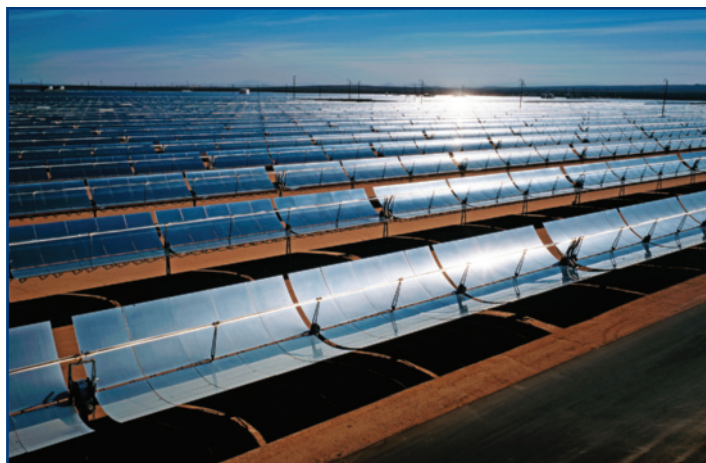
Figure 9.1: Parabolic trough solar collectors at Kramer Junction, California.
