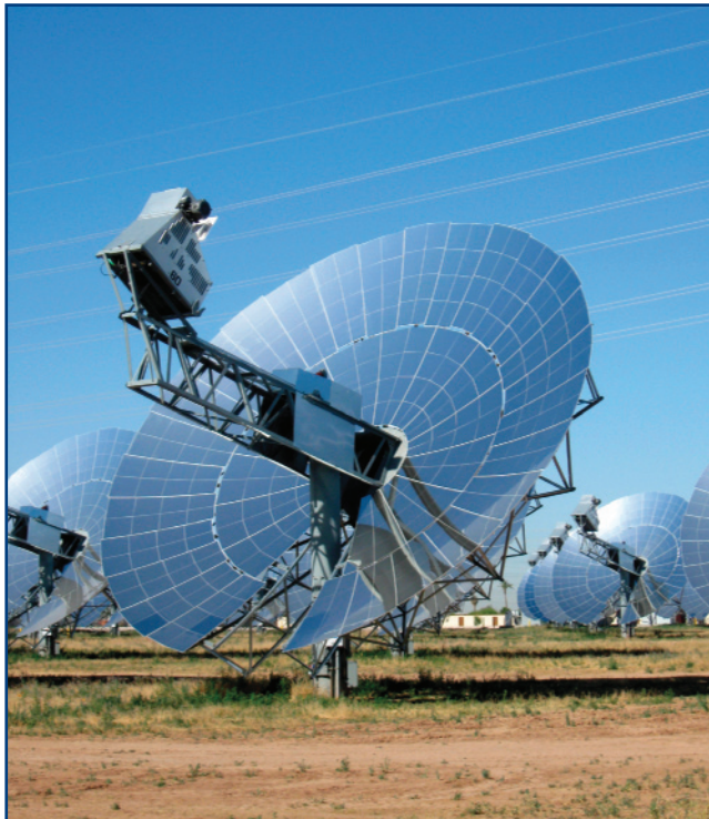
Figure 9.3: Parabolic dish solar collectors at Maricopa Solar Project in Peoria, Arizona showing the Stirling engine used to convert heat to mechanical energy.
